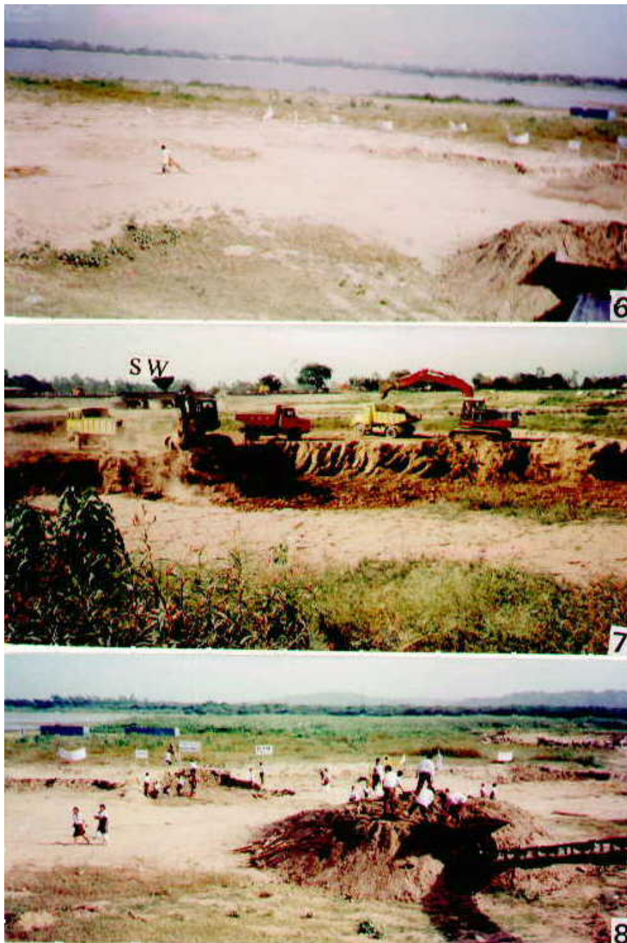
Figure 6. Manual desilting of the dried up portion of the Sukhna Lake bed. Peoples' effort 'Shramdan' has been mounted since 1988 for this purpose. The silt has collected towards the SW embankment. In the basin adjoining the Siwalik Hills there is still enough water though shallow (Photo June, 1993).
